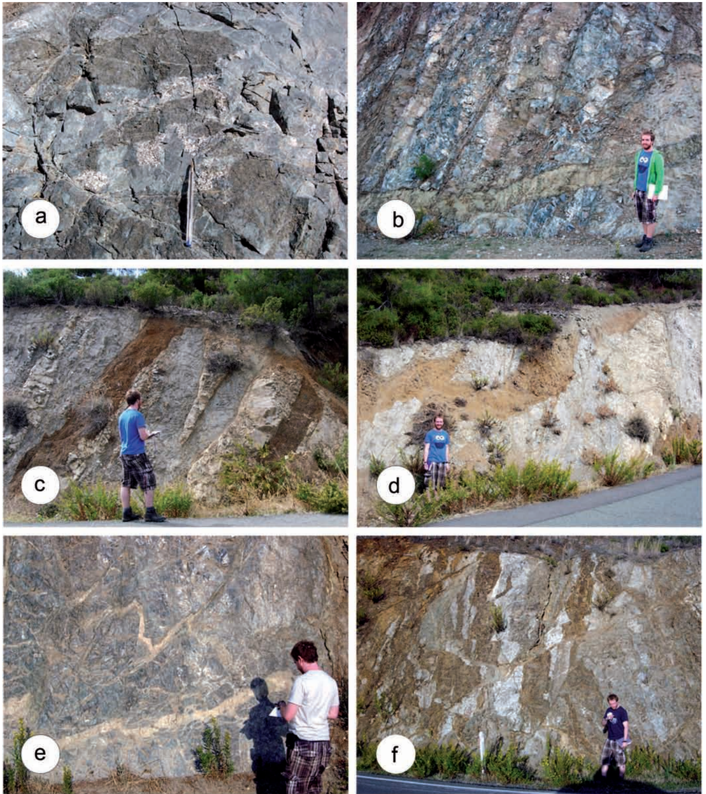
Fig. 16 - Field photographs of lithologies and structures along the road section studied to the north of the Arakapas Fault Zone. a- Small xenoliths of gabbro within grey sheeted diabase dyke; b- Typical grey sheeted dykes that are transected by a late-stage brown dyke at a low angle. Such relations indicate a complex rotation history; c- Classic outcrop (ideal for teaching), which shows early plagiogranite, cut by grey diabase dykes and then by brown diabase dykes. Towards the southern end of the transect (opposite a small blue industrial building); d- Irregular late-stage brown dykes cutting more steeply dipping grey dykes and plagiogranite, indicative of multistage rotation; e- Grey diabase dykes cut by small-scale listric extensional faults, which have been intruded by plagiogranite and re-faulted; f- Complexity of faulting affecting high-angle dykes. Plagiogranite is cut by grey dykes and then by brown dykes, which together are crosscut by planar extensional faults.
