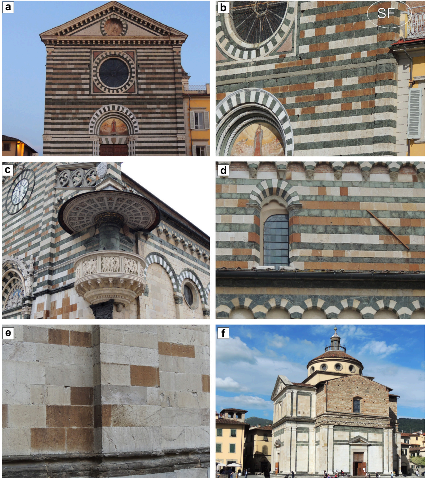
Fig. 1 - Religious buildings in Prato (Italy). a) Façade of San Francesco Church with ochre ashlars forming light bands alternating with the dark serpentinite. b) Detail of the San Francesco Church façade showing the ochre ashlars with a random distribution together with that having a linear distribution pattern. The white elliptic line indicates the location of samples (SF-4, SF-5). c) Santo Stefano Cathedral in Prato. d) Southern lateral aisle of Santo Stefano Cathedral in Prato displaying ochre ashlars displaying ochre ashlars according to a linear pattern with those aligned in the limestone layers one next to another. e) Detail of Santo Stefano Cathedral in Prato with a random ochre ashlar. f) Basilica of Santa Maria delle Carceri in Prato.
